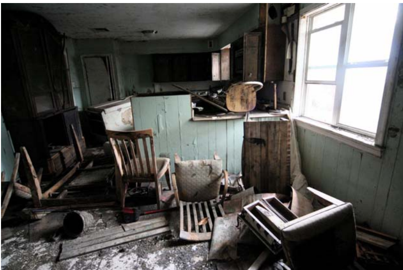
Destroyed remains of a home in the 9 th Ward.
